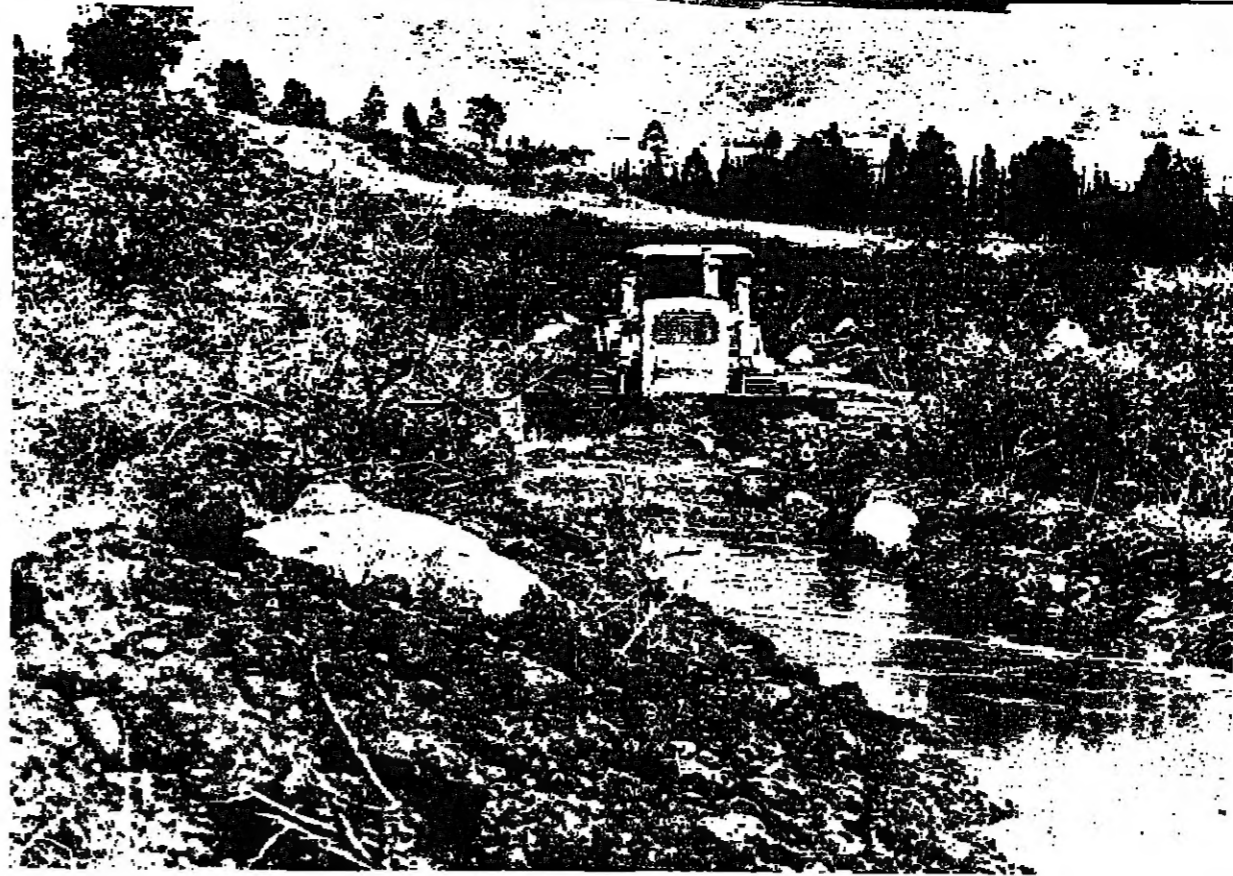
Nahal Sorek, depository of Jerusalem's sewage, is being widened and deepened. (Barzilay)
